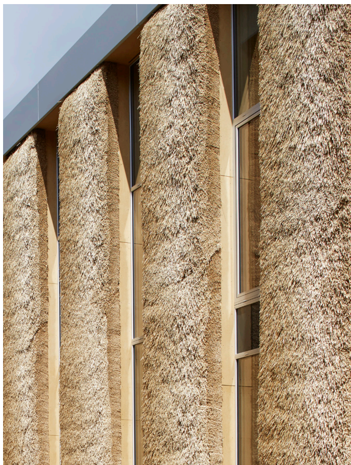
An example of local natural materials - Thatch Panelled Facade, The Enterprise Centre, UEA, Norwich
